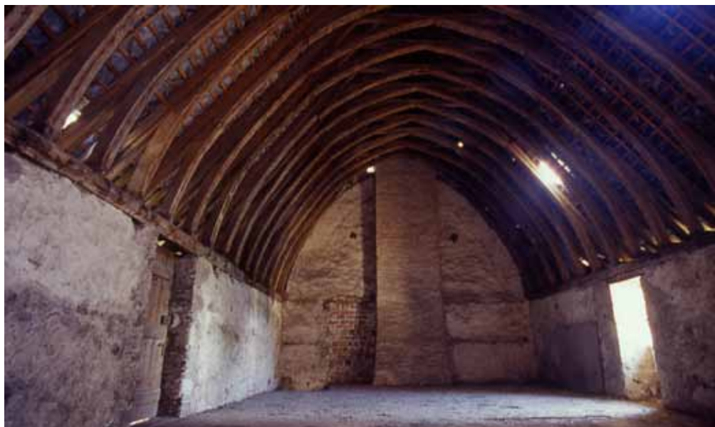
Framework of the refectory in the shape of an upturned boat hull. End of the 13 th century.
